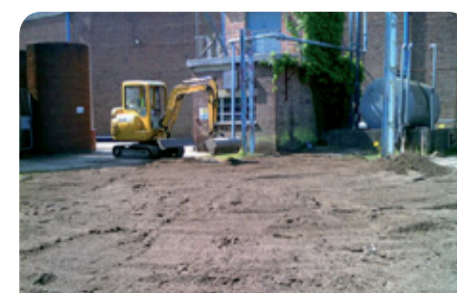
The former DARA site at Fleetlands following successful remediation
