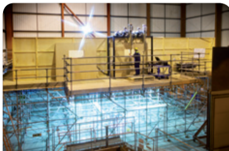
A mock-up of the room was constructed in NIS' high bay facility, to simulate the installation site
